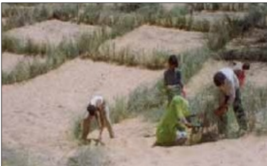
Fig. 4. People's participation in the preparation of checkerboard pattern on sand dunes in Bikaner and Churu district
