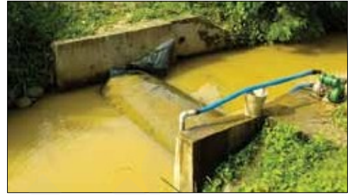
Fig. 1. Rubber dam at Chandesar-I, Khurda, Odisha
