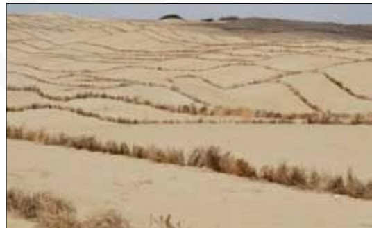
Fig. 5. Controlling sand slip over barren dune slopes using shrubs/grasses in horizontal pattern in Barmer-Bikaner districts
